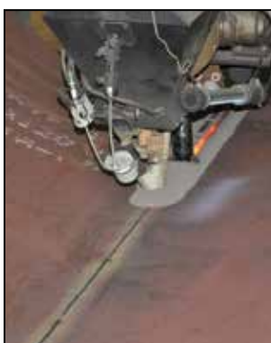
WELDING The can is then staged for longitudinal welding (Long Seam). During this process, the seam between the two plates is welded on both the inside and outside, using a tandem wire submerged arc welding process.
