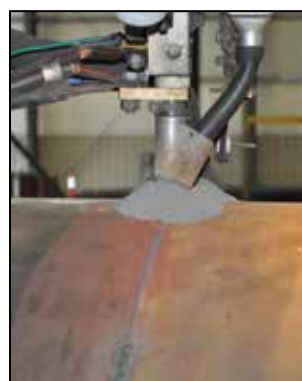
CIRCUMFERENTIAL WELDING During this last step of the manufacturing process, cans are fit together and the pipe is manufactured using the submerged arc process, according to customer requirements for specific lengths.
