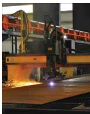
CUTTING A single flat sheet of steel plate is cut on a burning table, using plasma or cutting gases. This plate is cut according to the required width and length for the cylinder it will be rolled into.
