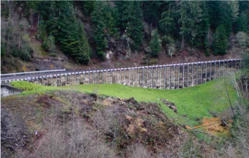
Completed Ground Stabilization Wall
