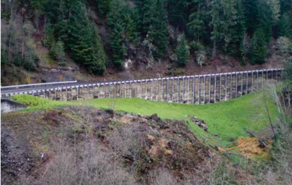
Completed Ground Stabilization Wall
