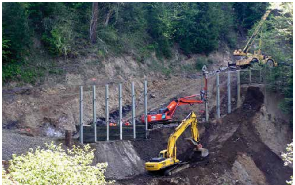
Construction of Soldier Pile Wall
