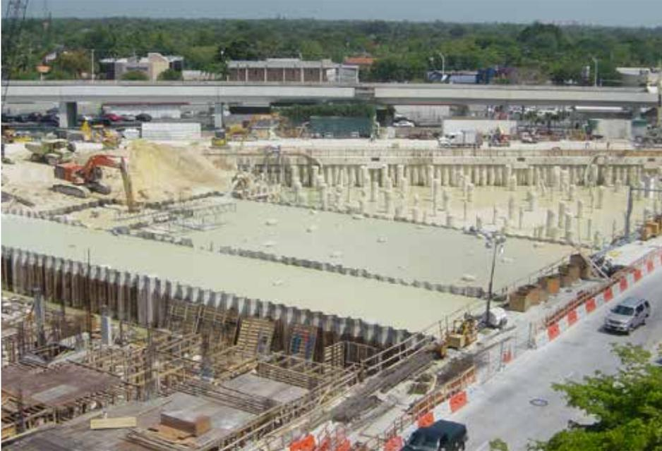
several sections reduced the concrete pour for the bottom slab into manageable sizes.
