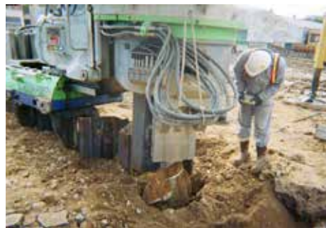
Installation of sheet piles
