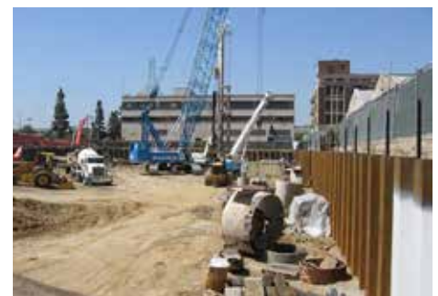
Excavation to P1 level
