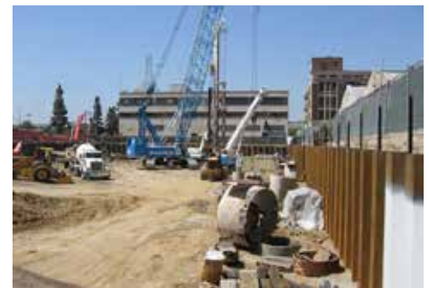
Excavation to P1 level
