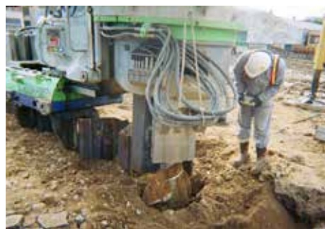
Installation of sheet piles
