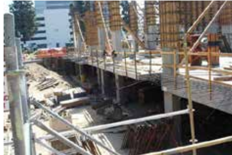
With P1 slab in place, construction proceeds upward in up-down zone
