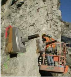
the drilling went deeper to get through the bedrock. Once the optimum drilling depth was found, a cementitious grout was pumped and the threaded bar inserted. When the grout cured, a hex nut was screwed down on the bar until the steel plate tightened against the rock face. Across the face of the bedrock, the post-tensioned force in the rock anchor system measured upwards of 620,000 pounds.
