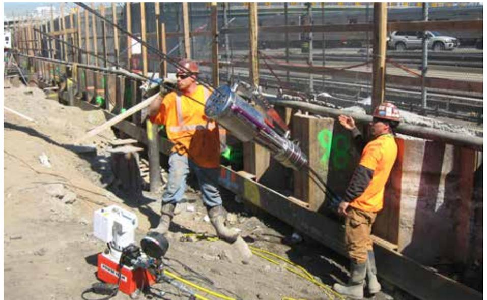
were ready for installation. Once installed and grouted, the anchors were stressed using Nucor Skyline's Smart Jack system. Even though there are variances in the unbonded lengths, this system uniformly distributes the stressing load to the grout bodies.
