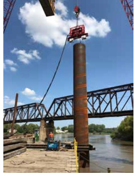
*Nucor Skyline produced 800 tons of 78" ID x .625 steel casings for a pier on the westbound I-70 bridge.
