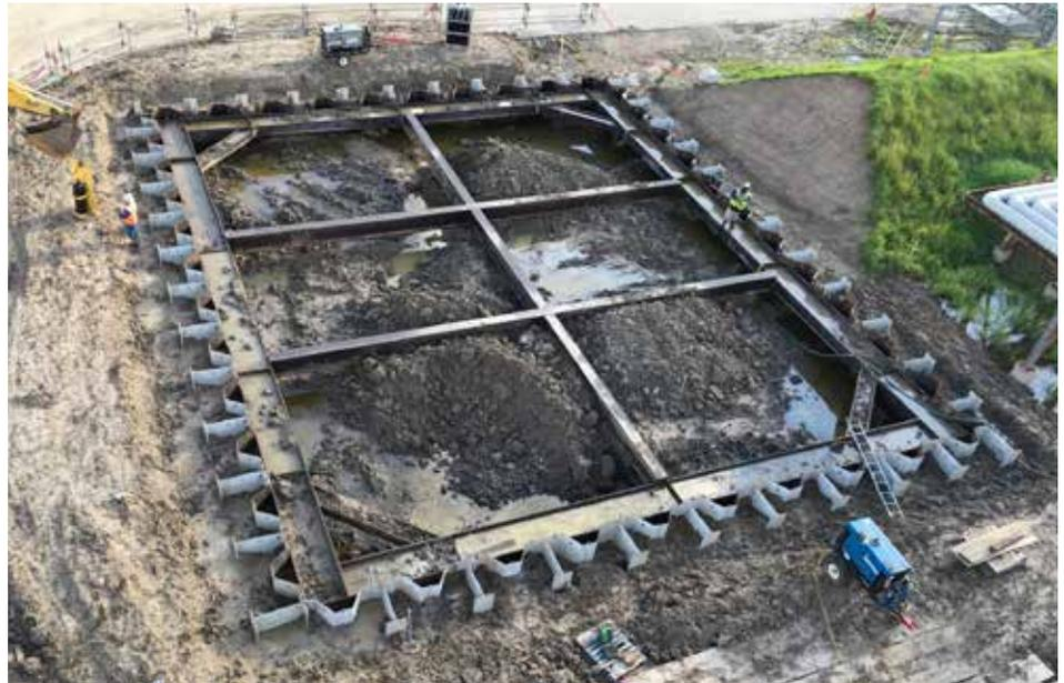
the cofferdam was to remain in place and act as the exterior form for the lift station.
