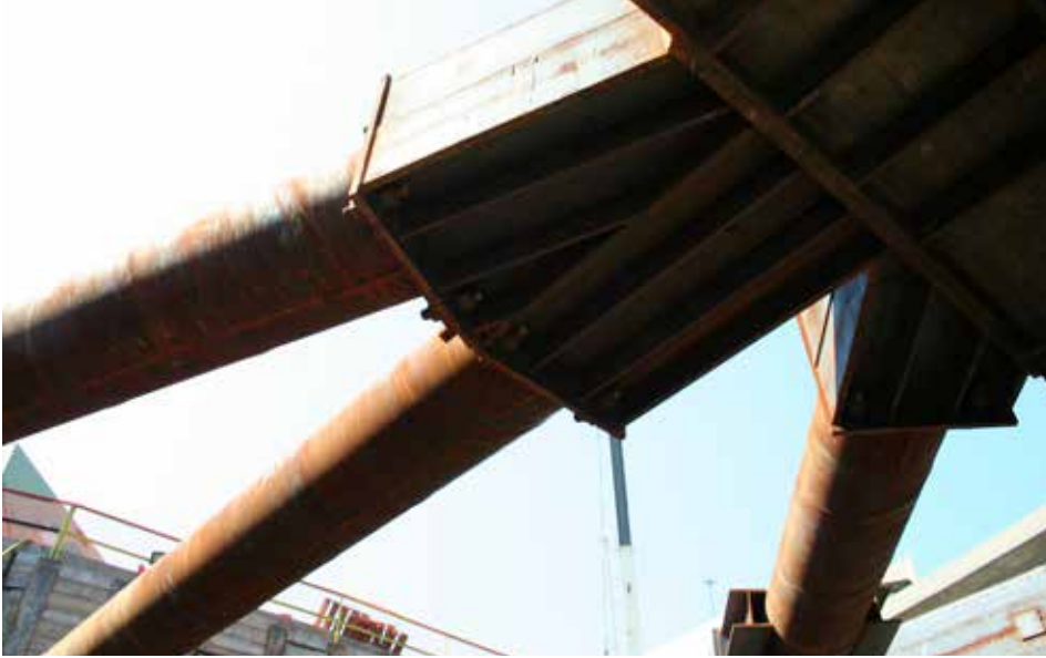
Fabricated pipe strut configuration
