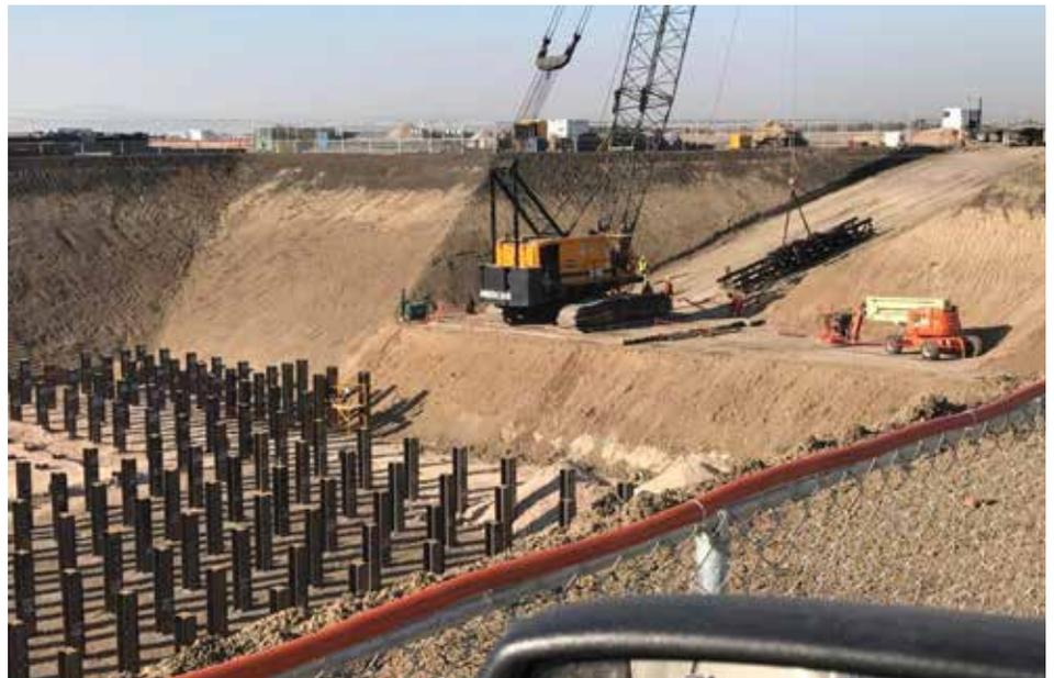
put into the ground. The design capacity of the piles was 135 tons in compression and 60 tons in tension, using HP 14x73 piles with a 70 feet embedment depth. This was one of the first jobs in this region to use steel piles instead of concrete.
