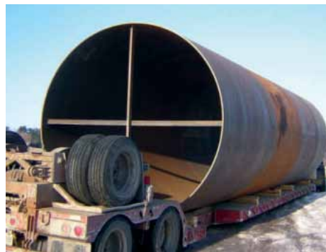
Steel casing being delivered to site
