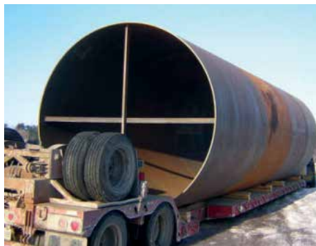
Steel casing being delivered to site
