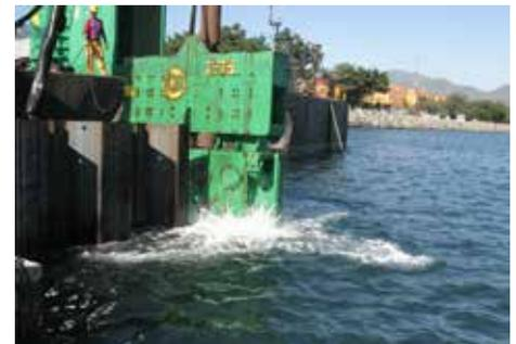
The next phase of the project adapted the existing structure of Band A, which was built in the conventional way with its base on slabs and the girders supported on reinforced concrete piles. Its original design operated at the dredging level of -12 meters (39 feet). The concrete structure of Band A was reinforced and a steel sheet pile system was constructed.
