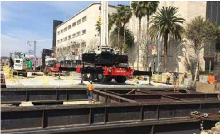
Wide flange beams used as bracing in the downtown excavation for the Purple Line Extension project in Los Angeles (Photo Credit: Skanska, Traylor, Shea JV)
