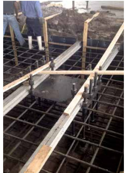
Threaded bar anchors nestled in spread footer reinforcement
