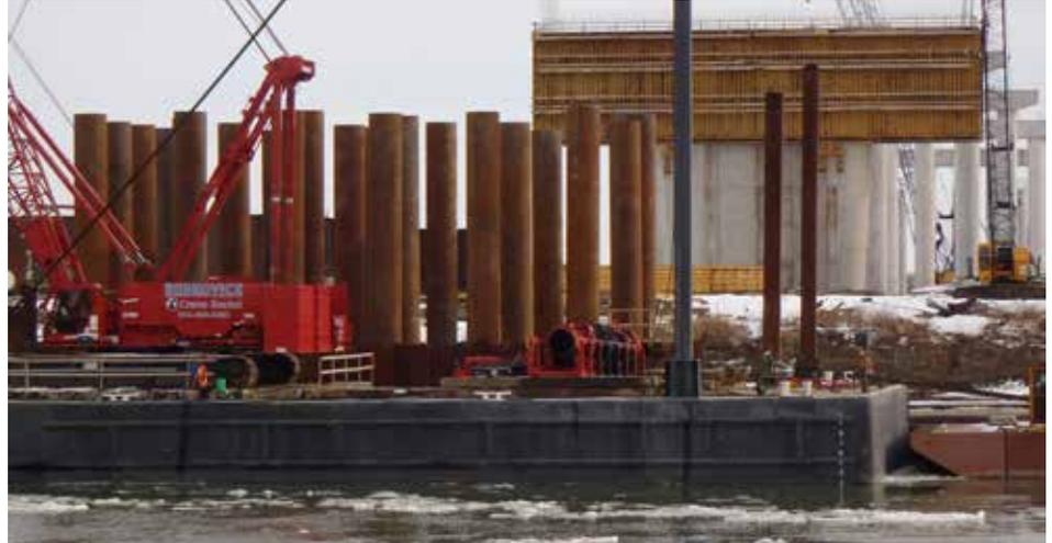
length for H-piles and concrete drilled shafts was too deep. Using pipe piles minimized the constructability risks for the river piers.
