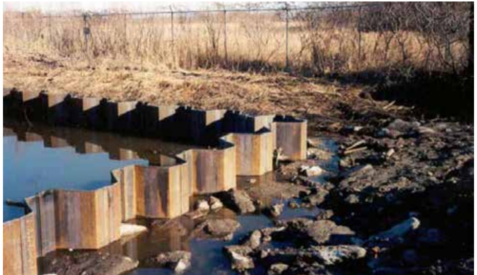
Above: Two walls of the cofferdam meeting before the closure piles were placed. Since good closure of the cofferdam was necessary the T-connection was fabricated on site.
