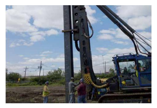
This project requires a driven pile foundation using HP 18 x 181 sections with pile tips driven to bedrock or stiff till, or drilled caissons to achieve the stiffness and load capacity specifications of the turbine manufacturers. A concrete pile cap of about 30 feet diameter at the tower base transfers the tower loads into the piles.
