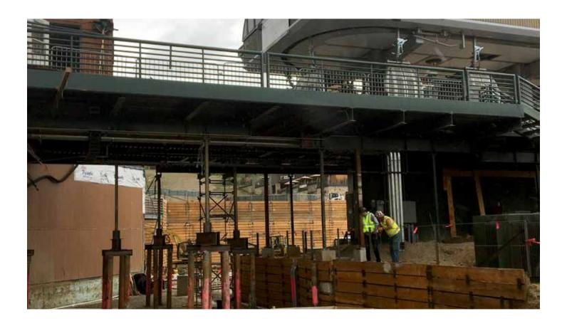
The Breckenridge Peak 8 Gondola project utilized 7.625" OD x .5" wall micropile casings beneath the mid-mountain base. Columns were then attached to the piles and used as temporary underpinnings during excavation.
