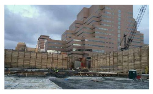
allowed the use of stock H-beam solider piles in lieu of utilizing heavier WF-beam sections from a mill rolling. Grouted hollow bar anchors were chosen for the tiebacks due to their speed and ease of installation. Nucor Skyline's large stock inventory of multiple H-pile sizes and 52mm and 40 mm hollow bar anchors allowed construction to proceed immediately after the contract was awarded.
