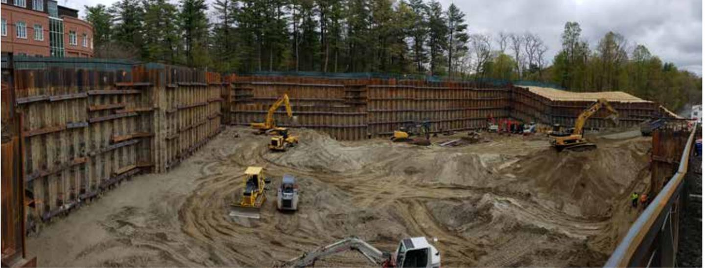
Nucor Skyline manufactured and shipped over length sheets directly to the site to avoid splicing sheets on-site. These 70-foot long sheets were cold-rolled and therefore, more economical and provided a cost savings over hot-rolled sheet piles. Multiple lengths of sheet pile were furnished, reducing the costs associated with extra steel on the project.
