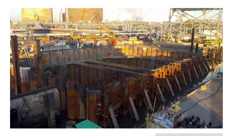
Pipe-Z wall constructed to form a cofferdam for a new fire water intake structure on the Delaware River in Marcus Hook, PA. The HP 14 x 89 were driven for foundation piles and were also installed as false work bracing for the pipe-Z cofferdam. Nucor Skyline's Engineering Department worked closely with Peirce Engineering in the design and sourcing of the material.
