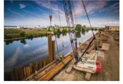
facility. The Nucor Skyline sheet piling had to be seal welded to assure water tightness. Dura-Bond Steel, of Export, PA, was able to set up a jig/bracing system which held the sheet pile pairs to the same width during the seal welding process. This allowed Ferraro to adjust their template, spacing their king piles correctly for the seal-welded pair of sheets.
