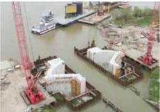
Nucor Skyline supplied sheet pile, H-pile, and pipe pile to build the new Empire Lock, located 40 miles south of New Orleans on the Mississippi River.
