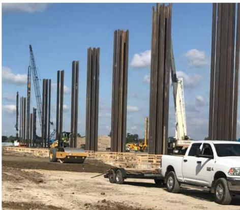
Auto parts supplier, Flex-N-Gate, is building a new 500,000 square foot manufacturing facility in Detroit, MI. Crawford Pile Driving installed Nucor Skyline's HP 12 x 53 pile, including tips and splicers for the project.
