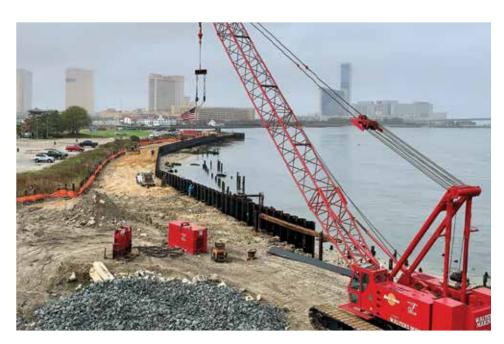
to delivery, the sheet piles were coated with 16mils Amerlock 2GF at 100% on both sides to extend their life in the harsher marine elements. The NZ 26 sheet pile, with the Larssen interlock, has one of the most watertight seals, making it ideal for marine use.
