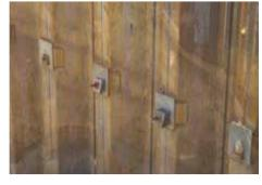
The contractor installed 50 linear feet of wall per day (a total of 1,200 linear feet was driven), a rate twice as fast as using slurry wall.
