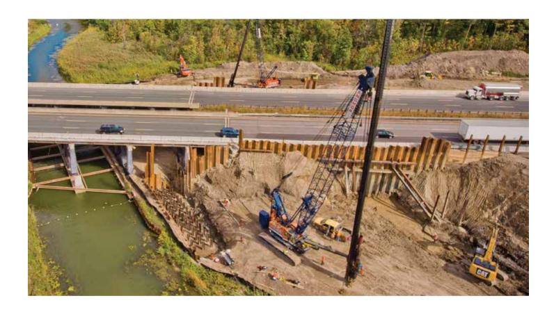
This project is part of the ongoing widening of Highway 400 to four lanes from Toronto to Barrie, Ontario. Widening of the existing Highway 400 bridge required foundation piles and shoring of the existing roadway to allow for bridge construction to be completed in two stages.
