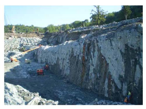
extensions, and tailrace to carry the water. Clearing each of the individual areas required extensive blasting through hard bedrock, as well as a support system to stabilize the slope and prevent future failures as large volumes of water flow down the Susquehanna through the power facility.
