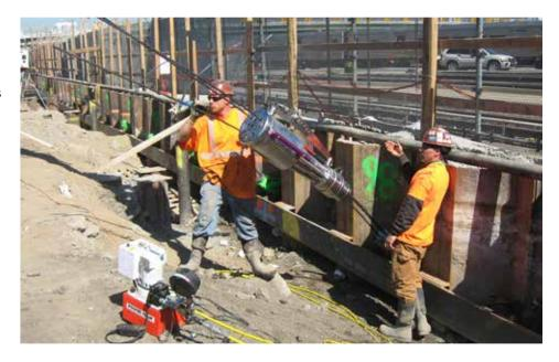
were ready for installation. Once installed and grouted, the anchors were stressed using Nucor Skyline's Smart Jack system. Even though there are variances in the unbonded lengths, this system uniformly distributes the stressing load to the grout bodies.
