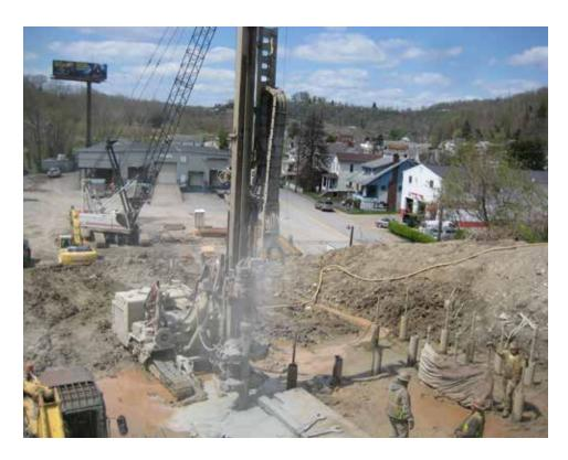
Micropiles are ideal for complex sites where low noise levels or low vibration is required, or where limited access such as low headroom and drilling is difficult. Additionally, when there are obstructions, large cobbles or boulders, high groundwater conditions, karstic rock, or nearby sensitive structures, micropiles are the right product for the project. The unique characteristics of micropiles make them a perfect solution when other deep foundation methods are not suitable.
