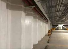
also increased available parking space, because the sheet pile could be driven to the perimeter of the property, maximizing all available space. And with the welded interlocks of the Z-shaped sheet pile, the wall is watertight.
