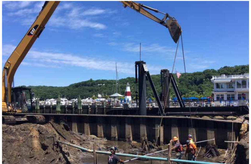
The seven-foot tide change gave workers a small window to install the tie rods. The threaded bar and walers were used in combination to tie the bulkhead wall to the deadman wall. Installation could only be accomplished at the mid-point in the tidal range during daylight hours.
