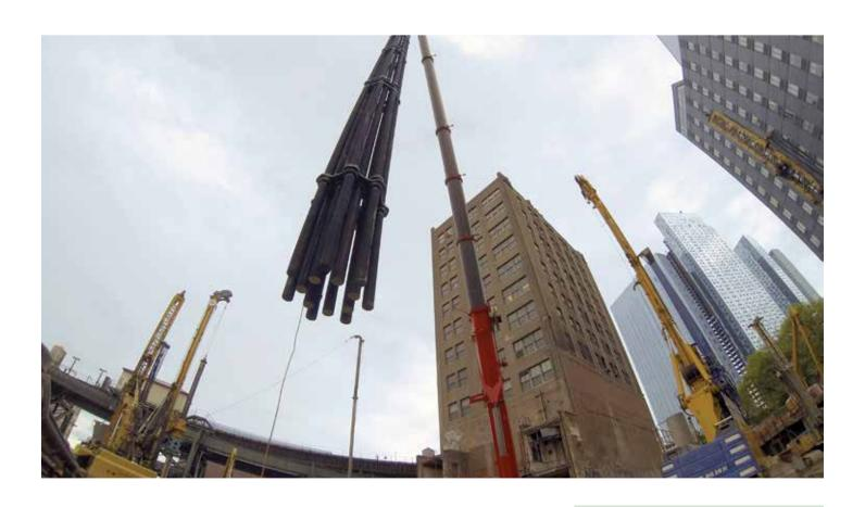
Queens Plaza Park is slated to be the tallest residential mixed used high-rise in Queens, NY. The 978,000 sq. ft. tower will be constructed over 900 ft. tall. The foundation piles consisted of 90 drilled shafts containing over 1,000 tons of #28 Gr. 75 threaded bar cages fabricated by Nucor Skyline's Camp Hill, PA facility.
