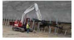
sub-surface conditions. Nucor Skyline provided R38 hollow bar anchors, totaling over 4,200 galvanized, 3-meter bars. The design load of the hollow bar piles was 13.6 kips and was tested to 27.2 kips.
