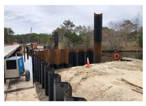
on many projects in the past. Moffat & Nichol suggested using the sheet piling as there was very limited right of way while building the temporary bridge. The sheet piling was used to support the temporary access as the bridge was built.
