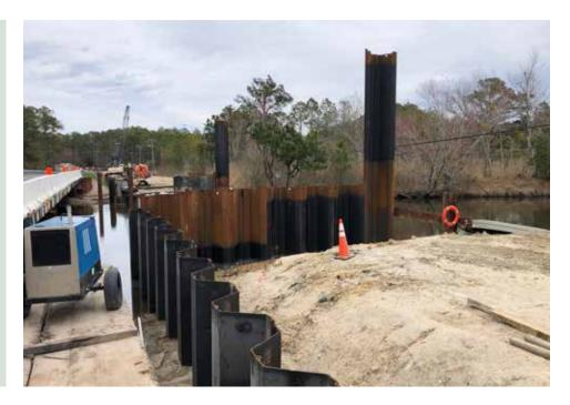
suggested using the sheet piling as there was very limited right of way while building the temporary bridge. The sheet piling was used to support the temporary access as the bridge was built.
