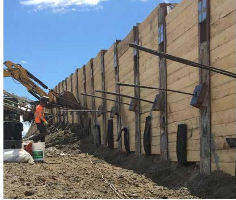
The end of the line ground anchor wall of the Southeast Rail Extension (SERE) Light Rail project is approximately 16,000 square feet long, and includes the installation of over 40,000 LF of strand tiebacks, ranging in length from 57' to 76'.
