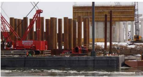
length for H-piles and concrete drilled shafts was too deep. Using pipe piles minimized the constructability risks for the river piers.
