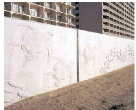
sheet piles (28-foot lengths) supplied by Nucor Skyline. The main wall is cantilevered in some sections, and in others, anchored to a secondary wall of Z-shaped sheet pile. According to Roehrs, the design would protect against a 9-foot surge and “survive a 1-in-146-year storm.”
