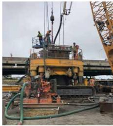
equipment needed to build a new three-lane northbound structure. Crews from Condon Johnson & Associates will drive Nucor Skyline 118" and 71" OD pipe piles into the ground between the existing bridge and the temporary construction bridge. Once the bridge piers are in place, the new bridge deck can be built on top of them.
