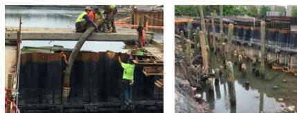
The Wynn Casino in Everett, MA needed a sheet pile bulkhead wall to be built for their water shuttle facility. Multiple sizes of Z-shaped sheet piles, as well as cold-formed threaded bar, helped complete the project.
