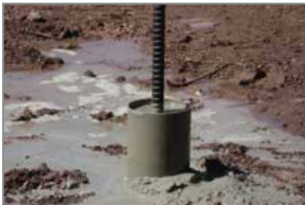
Micropile casing installed with fully threaded 75 ksi bar reinforcement
